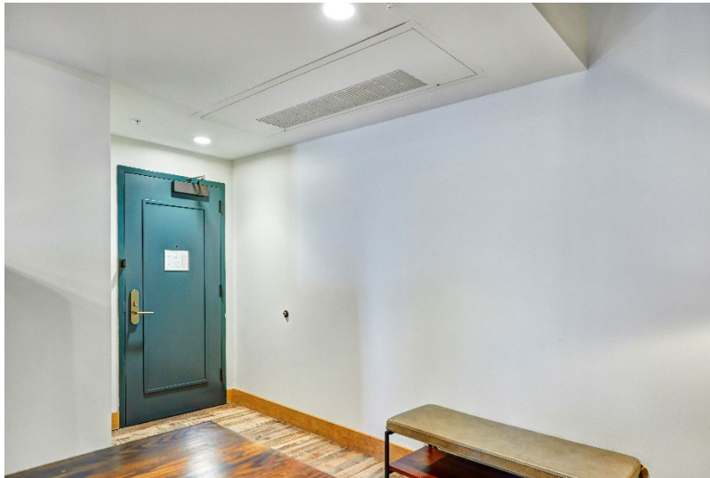
The Williams Comfort Products IPS fan coil units are concealed within the ceiling of guest rooms and common areas.
