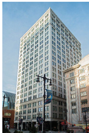
The Atlantic, a 200-year-old building in Philadelphia that now features 228 apartments and LEED Gold certification.
