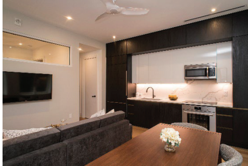
Long, slim duct registers on the ceiling are the only visible evidence of The Atlantic's unique Williams Comfort Products IPS fan coil system.
